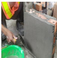
Gambar 3. 33 Plesteran Dinding Bata
